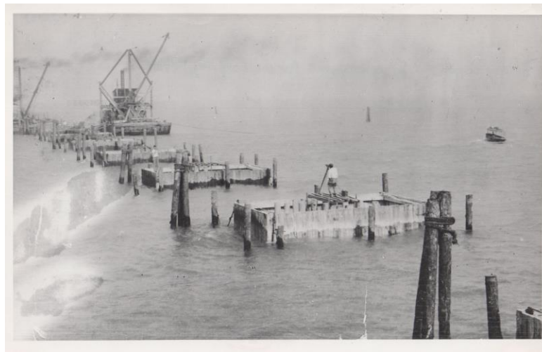
Black and white photograph taken during the construction of cofferdams in order to build concrete piers for the Long Key Viaduct on the Overseas Railway.
