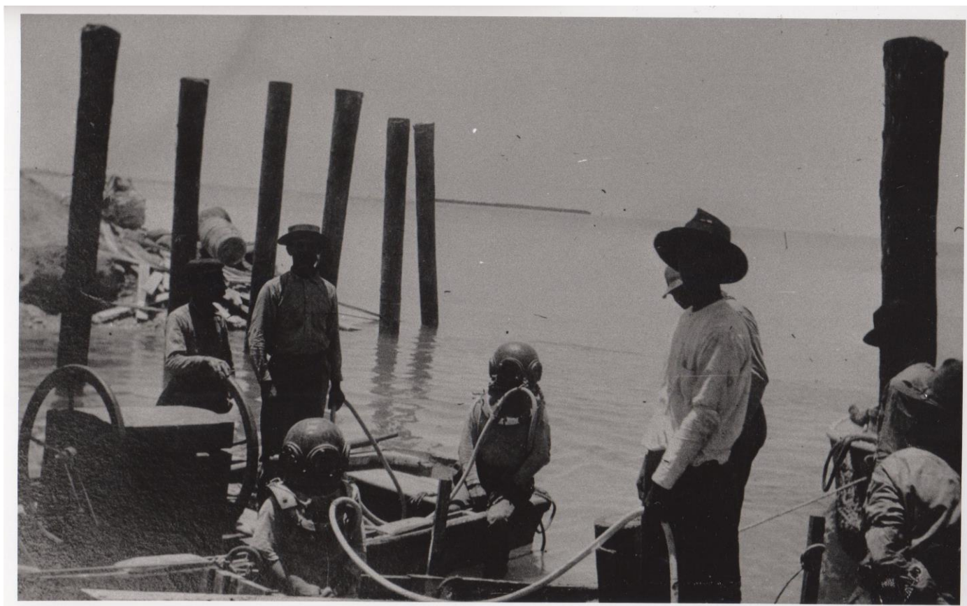
Black and white photograph of hard hat divers working on the bridge piers for the Florida East Coast Railway Company.
